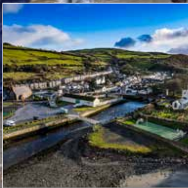
Glenarm Visitor Information Centre, Glenarm Marina, 16 New Road, Glenarm BT44 0AP
